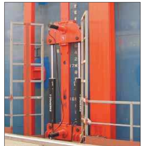
▼ Each climbing unit consists of two 70 tons double-acting cylinders and two 20 tons locking cylinders.
